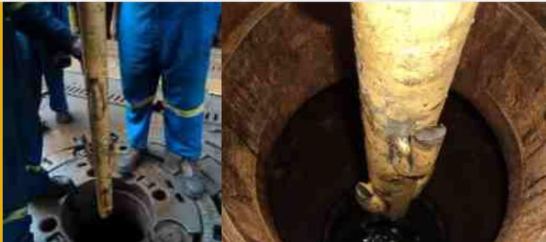
*Global ETC is experienced at managing fishing situations when debris or pipe gets stuck in the wellbore. The key elements of a fishing operation include an understanding of the dimensions and nature of the debris to be removed, the wellbore conditions, the tools and techniques employed and the process by which the debris will be handled at surface.*
